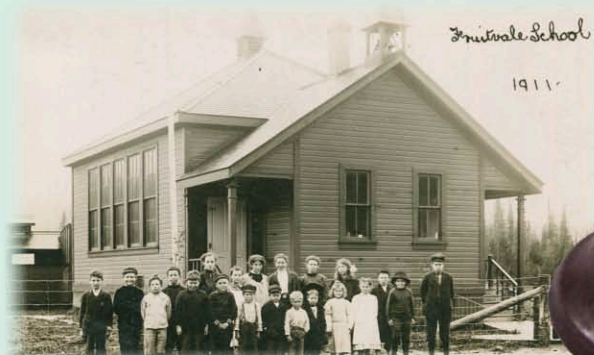
This beautiful new school, Fruitvale's second, opened in 1910, serving as the community hall as well.
